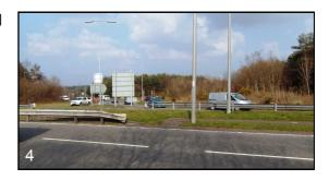
Provision to make the Pontarddulais Cross (A48/A4240 junction) roundabout safe for cyclists would be needed. This would likely involve tightening the curvature of the entry lanes to slow traffic.
