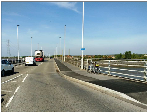
Widened footway on N. side of bridge.
