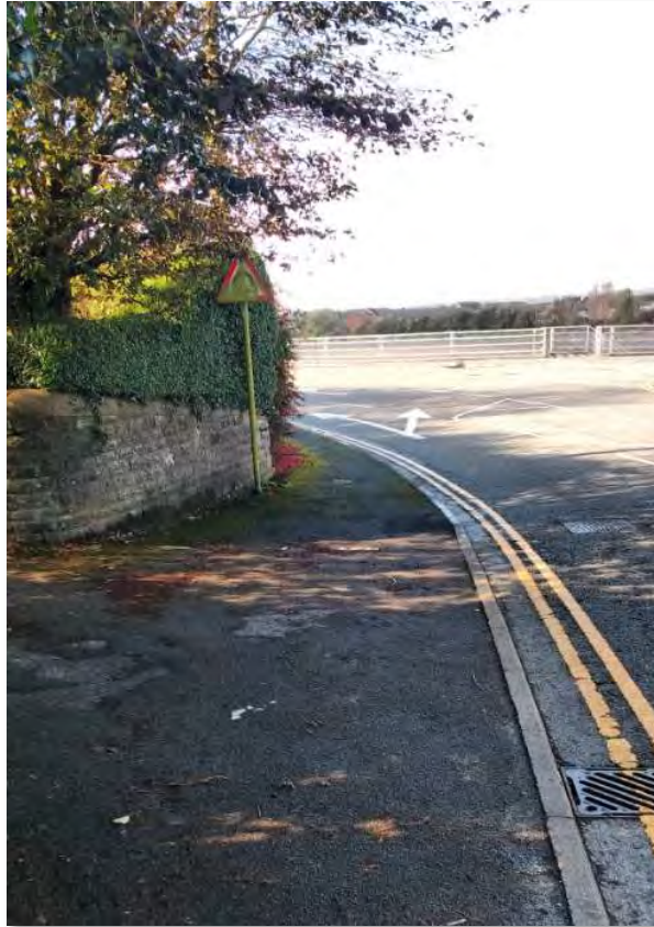
Photo showing visibility approaching crossing point
