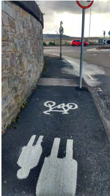
Photo showing narrow width of existing cycleway
