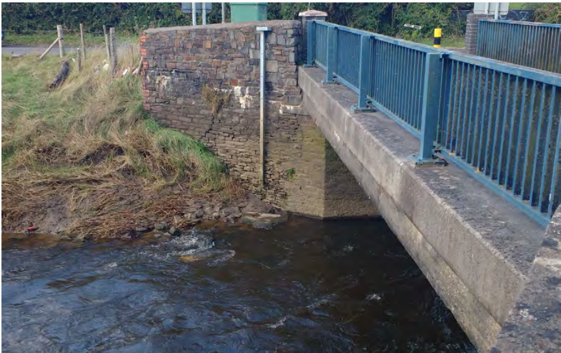
Photo – West Abutment of Island Bridge
