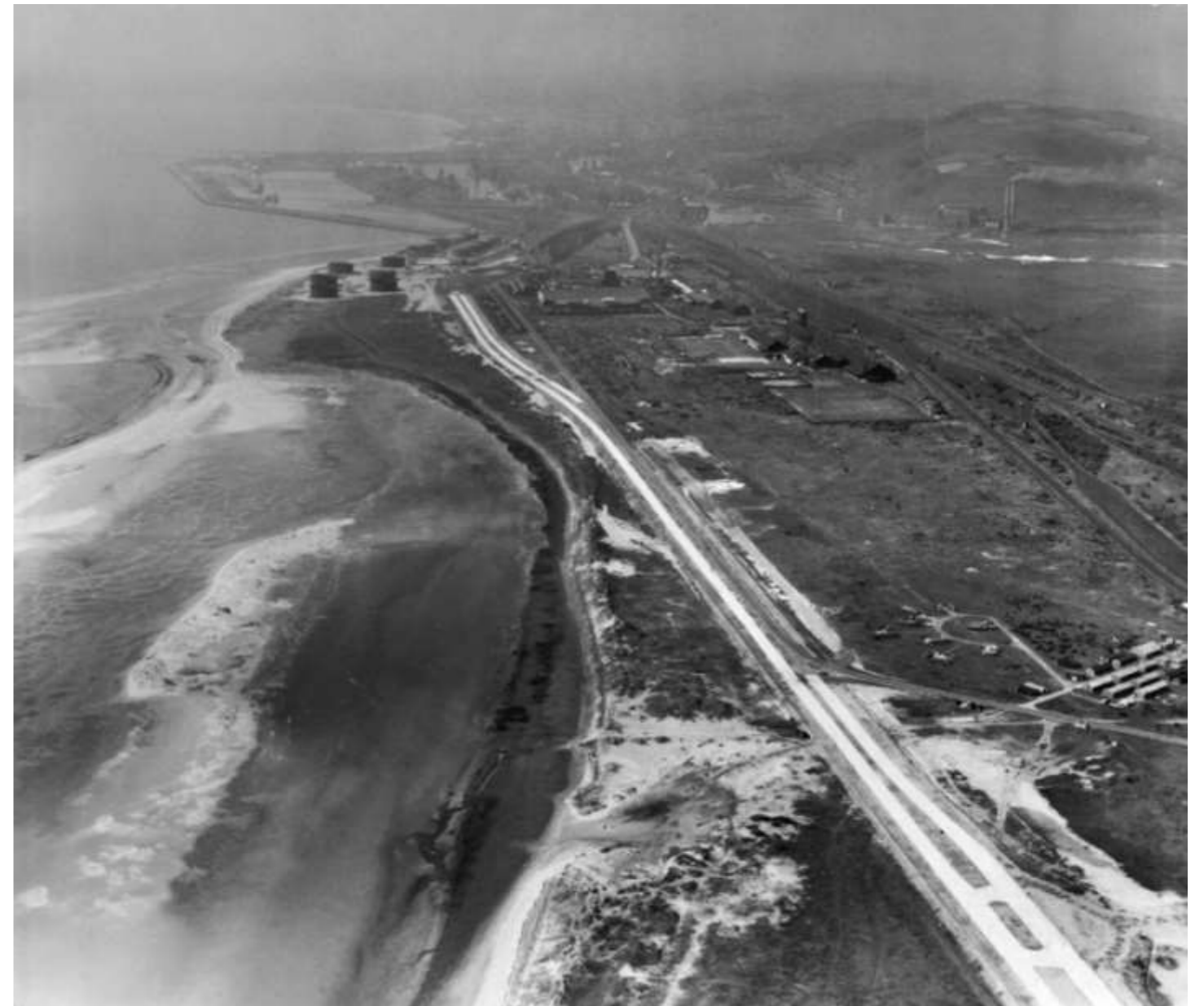
Fabian Way, or Jersey Marine Road, now A483, was constructed between May 1946 and September 1950. Amazon now lies to the right of the dual carriageway and the bay area was reclaimed for petro-chemical tanks, now the Swansea University Bay Campus. (image courtesy of the RCAHMMW)
